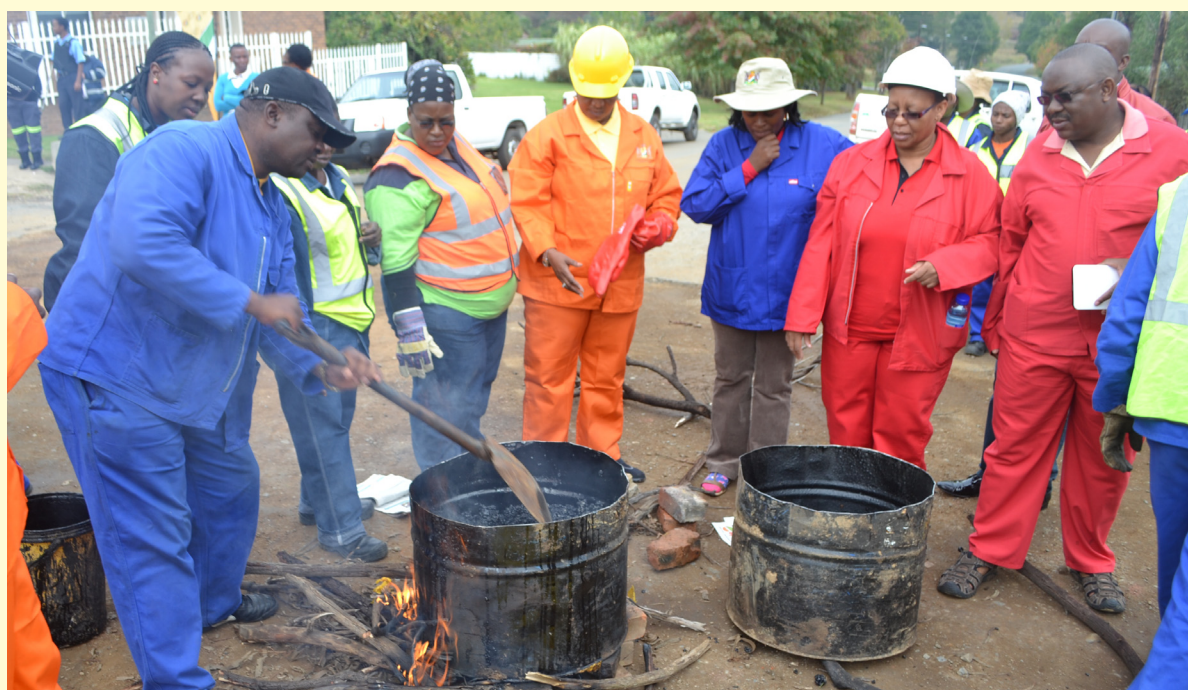
Officials melting material used to patch potholes
