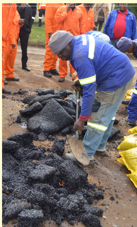
A road worker hard at work patching potholes.
